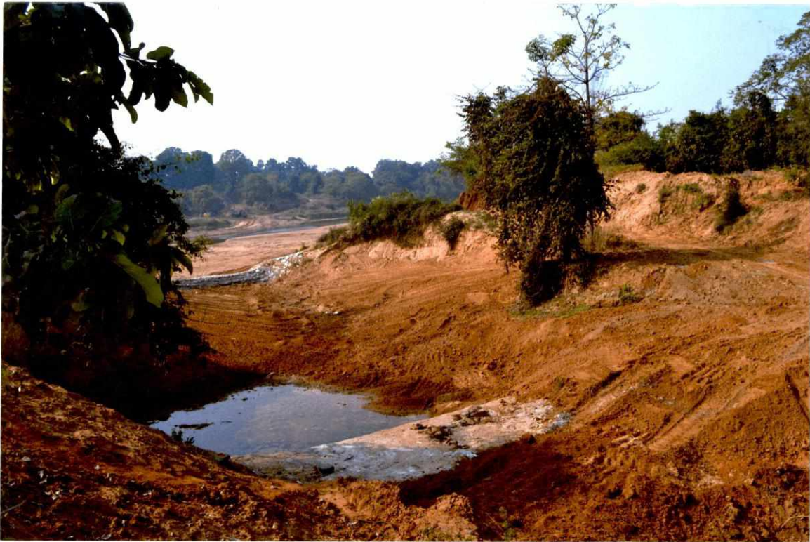
Photo 12: Check dam in the nallah
